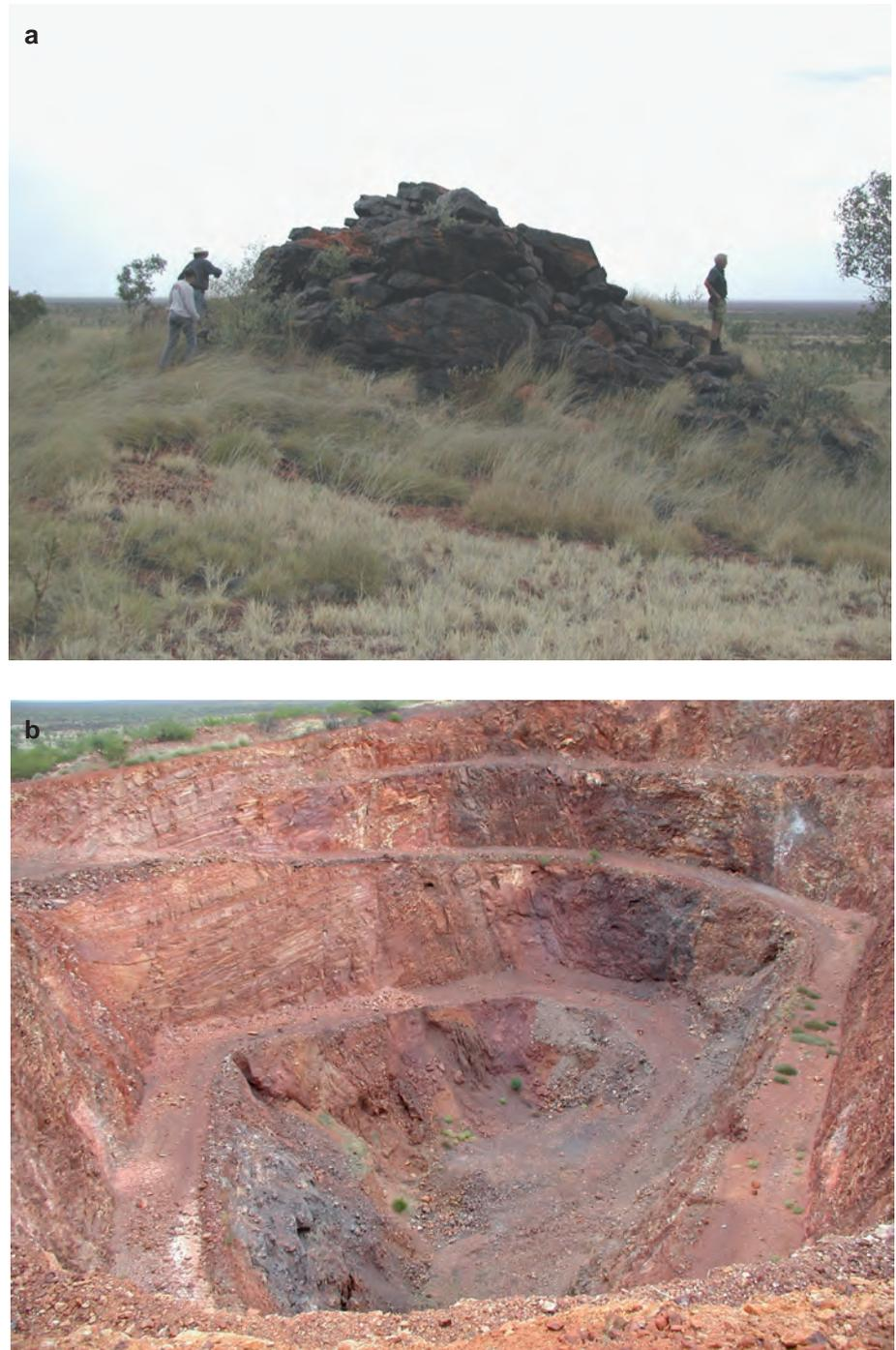
**Figure 60.** Eldorado mine, Tennant Region. (a) Surface expression of ironstone body and (b) ironstone (darker tone) within open pit.
